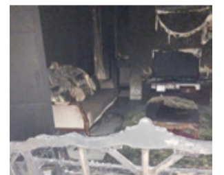
The gutted house.
